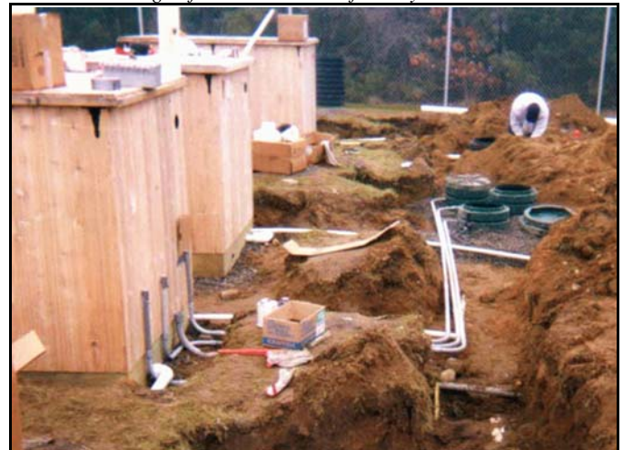
Waterloo Biofilter during installation (3 side by side installations)
