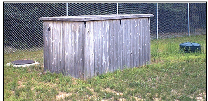
One unit, after installation.
