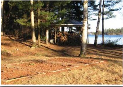
**Figure 4. Multiple-barrier Waterloo “flat bed” and shallow area bed system protecting sensitive lakefront property — as simple and aesthetic as a filter bed, but with an underdrain to promote free-draining aerobic conditions and a maintenance contract for sustainability.**
