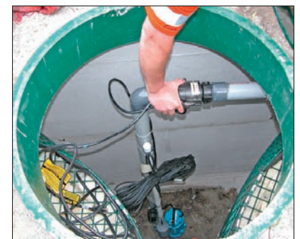
Above, (from back to front) Mike Pauze, Allan Lalonde, and Kirk Hastings set the bottom of the biofilter container tank. At right, a technician secures the quick disconnect for discharging and recirculating the treated effluent.
