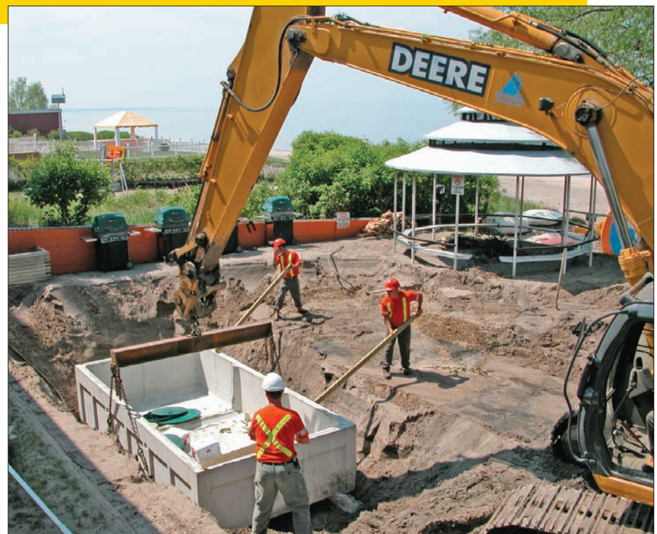
Above, (from back to front) Mike Pauze, Allan Lalonde, and Kirk Hastings set the bottom of the biofilter container tank. At right, a technician secures the quick disconnect for discharging and recirculating the treated effluent.
