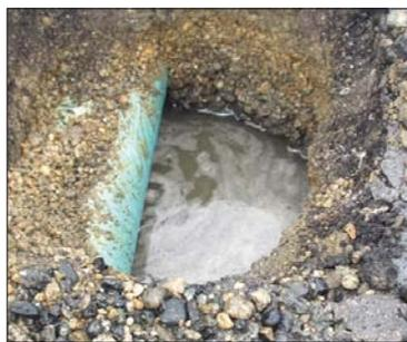
**Wastewater stands in the failed pressure distribution disposal field.**
